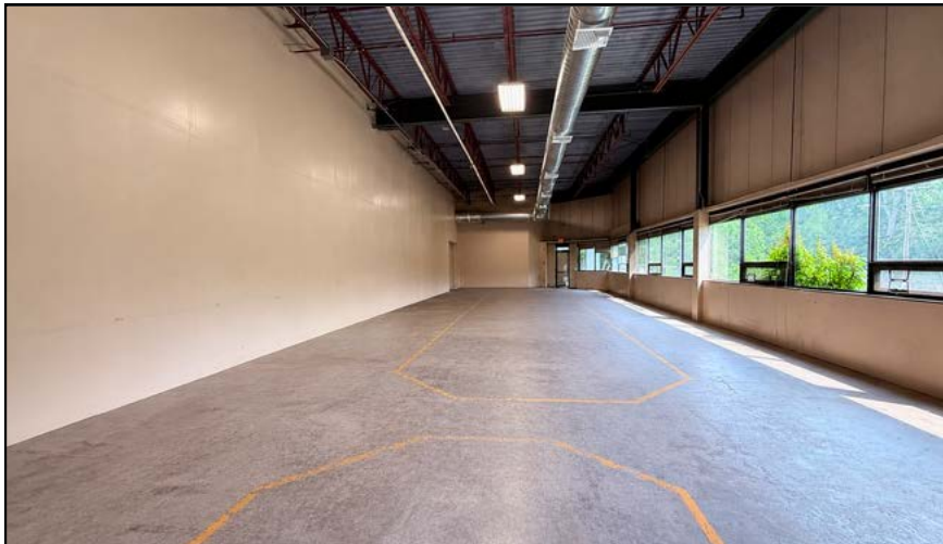
CENTRAL AIR-CONDITIONED FLEX SPACE WITH A 16' 7" CEILING HEIGHT (TO STEEL)
