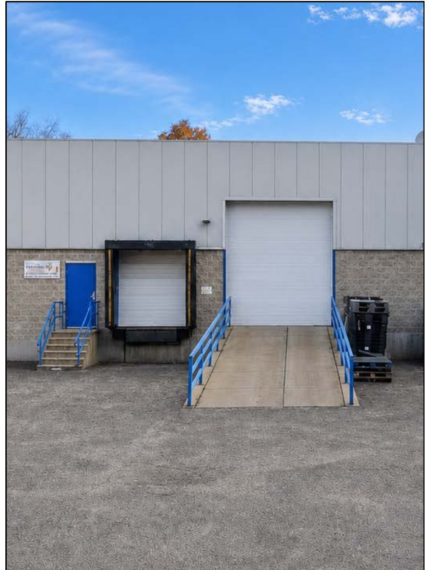
ONE 8' W X 10' H LOADING DOCK WITH BUMPERS AND LEVELER & ONE 12' W X 14' H DRIVE-IN DOOR WITH RAMP
