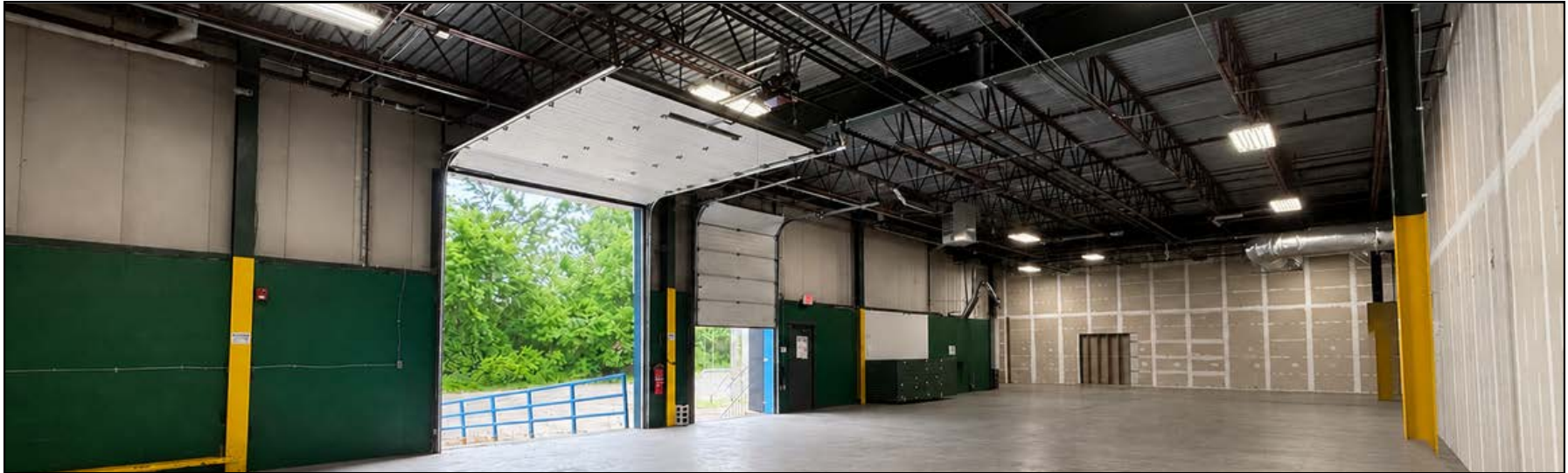
OPEN WAREHOUSE SPACE FOR LOADING WITH ONE ENTRY DOOR AND A 16' 7" CEILING HEIGHT (TO STEEL)
